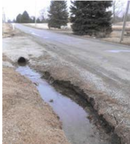
FIGURE 4 – Lutz Road Ditch
