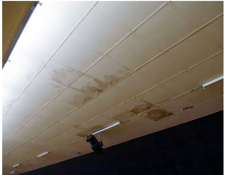
The photos on this page illustrate interior water damage inside of the vacant AMF Circle Lanes, bowling alley. (1225 Holiday Drive)
