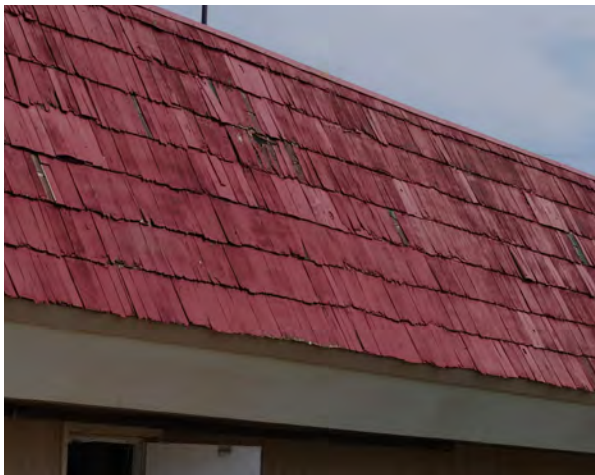
Left & Right: Deteriorated wood shingles on the roof of Kep's Country Kitchen. (506 IAA Drive)
