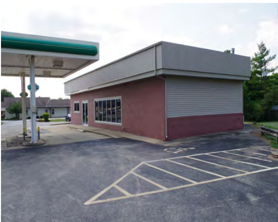
Left: A vacant former filling station. (1220 Towanda Avenue)
