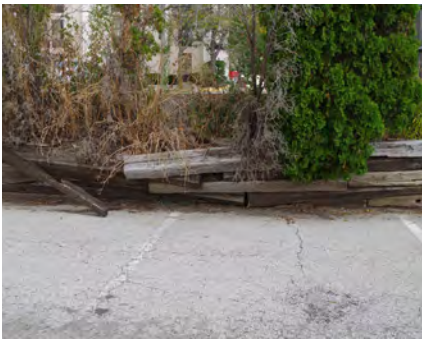
Above: The parking lot and retaining wall in the rear of the vacant K-Mart are deteriorated. (1608 East Empire Street)
