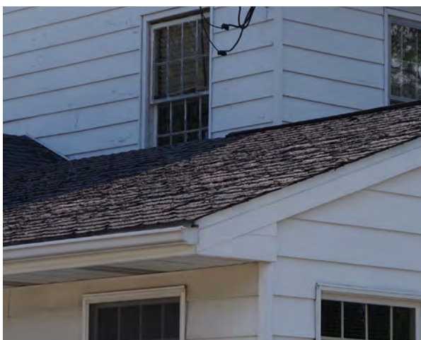
Left: The shingles on this vacant home, that has been converted into an office, are deteriorated. (1234 Empire Street)
