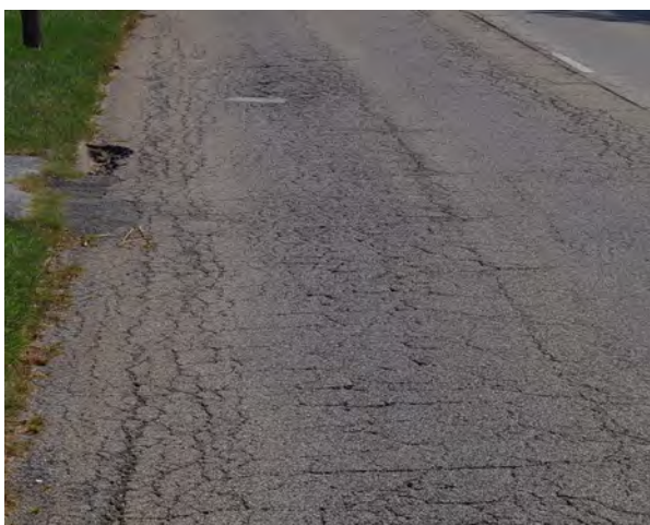
Left: The street pavement along Empire in front of Bloomington High School is deteriorated.
