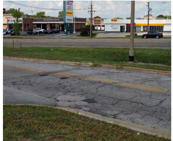
Left: The curve transitioning IAA Drive from north-south bound orientation to east-west is deteriorated.
