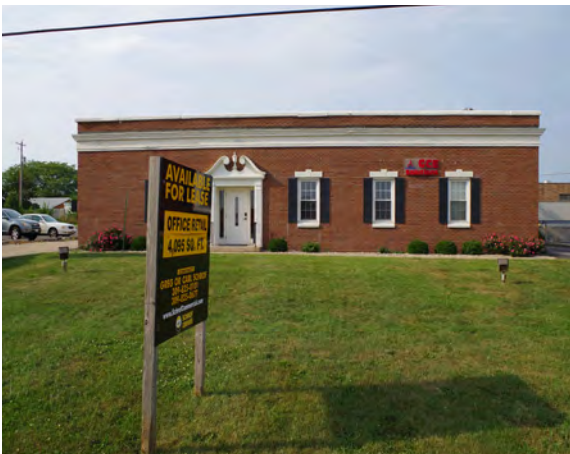
Left: A partially vacant office building. (1408 East Empire Street)
