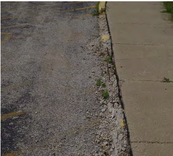
Above: Deteriorated curbing on the lot of the former bowling alley. (1225 Holiday Drive)
