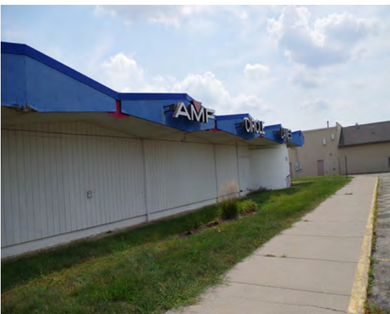
Left: The vacant former AMF Bowling Alley. (1225 Holiday Drive)
