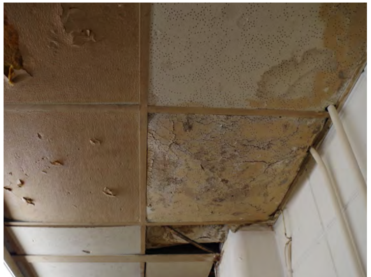
The photos on this page illustrate interior water damage inside of the vacant AMF Circle Lanes, bowling alley. (1225 Holiday Drive)
