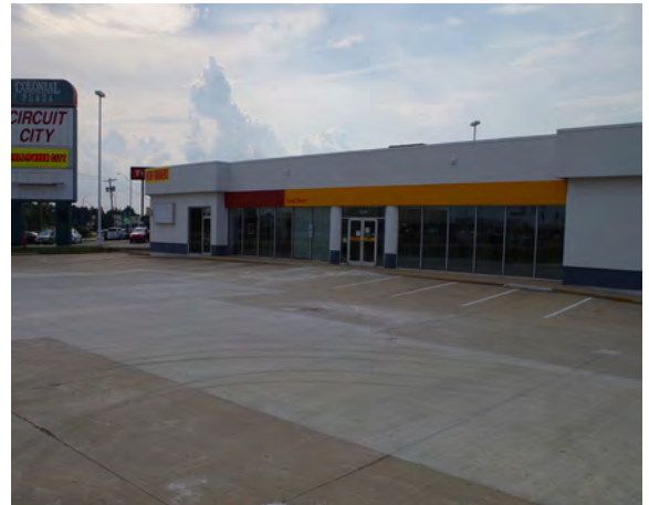
Right: A vacant former filling station. (1504 East Empire Street)
