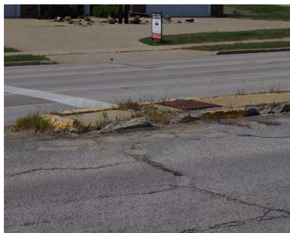
Left: The street pavement along Empire in front of Bloomington High School is deteriorated.
