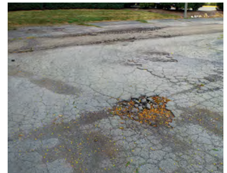
Below: The parking lot for Cash Loans on Car Titles is deteriorated. (604 IAA Drive)
