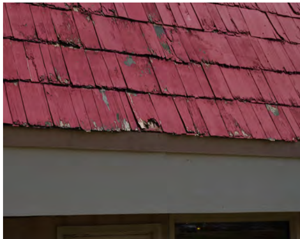
Left & Right: Deteriorated wood shingles on the roof of Kep's Country Kitchen. (506 IAA Drive)
