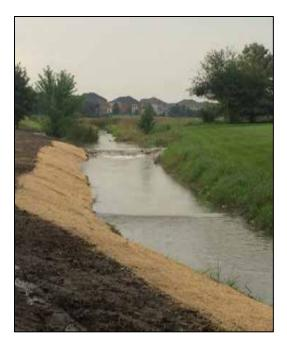
Continued residential development in a neighborhood east of Hershey Road caused a stormwater stream to be redirected. The stream eventually was running atop an exposed sanitary sewer. In summer 2014, Public Works relocated the portion of sewer away from the stream. It then installed stone "riffles" in the stream. Riffles slow down the speed of water, thereby allowing for sediment to drop and reducing erosion of the banks.
