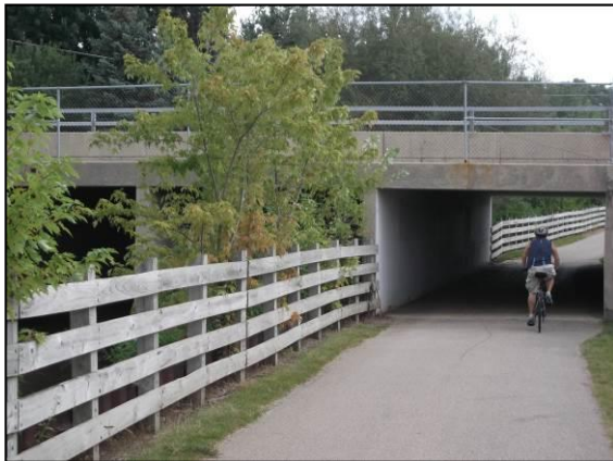
Figure 4.8. Trail underpass of Hershey Road.
