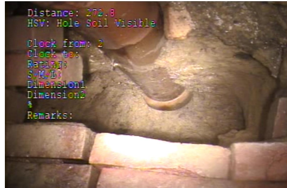
Holes in the Douglas Street Sewers filmed by CCTV
