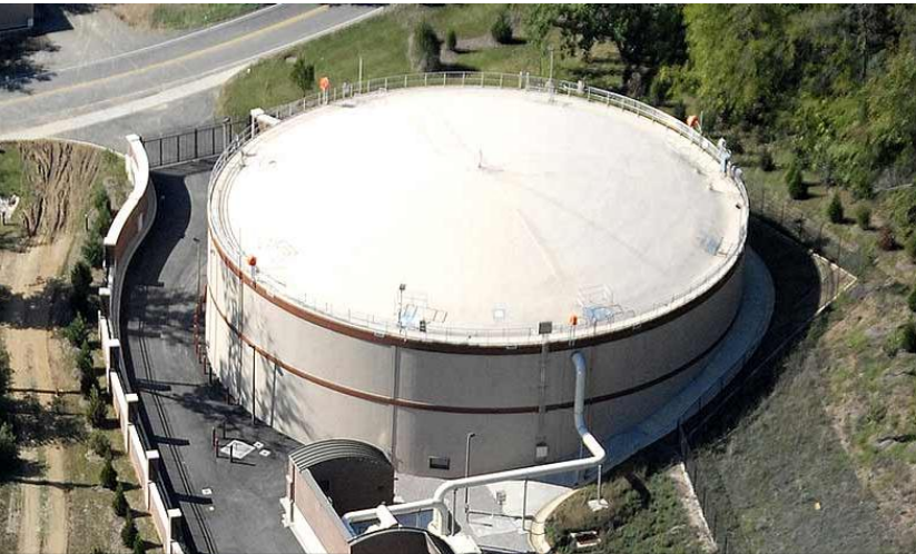
Wastewater storage facility, Knoxville, Tenn.
