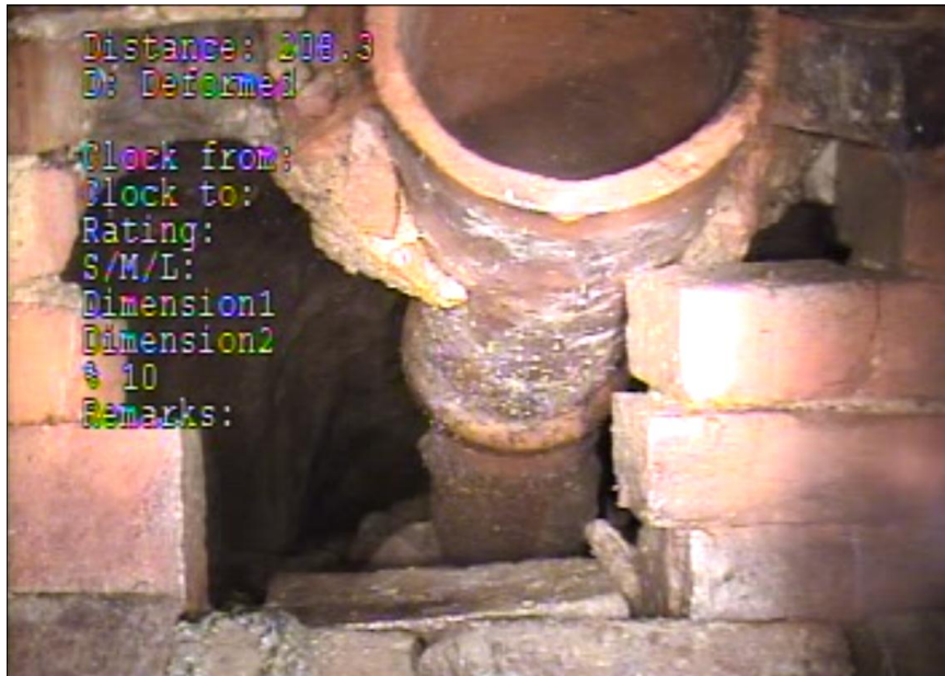
Holes in the Douglas Street Sewers filmed by CCTV
