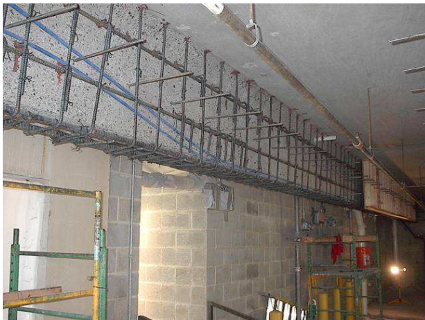
Placement of Mild Reinforcement and PT Cables
