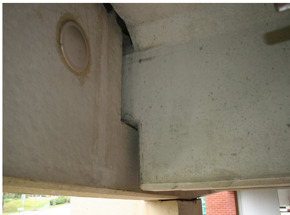
Dapped End at Spandrel Beam
