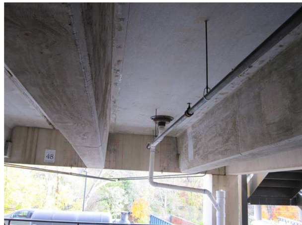
Completed Concrete Enlargement of Double-Tee Stems
