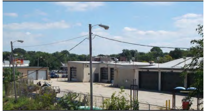
The 'Bus Barn' from South Main overpass.
