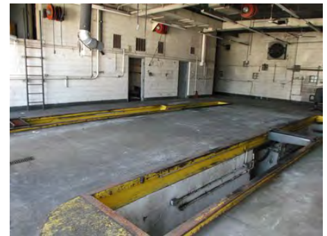
Vehicle maintenance bays.
