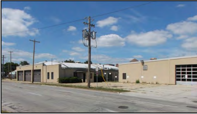
The 'Bus Barn' from East Oakland Avenue.
