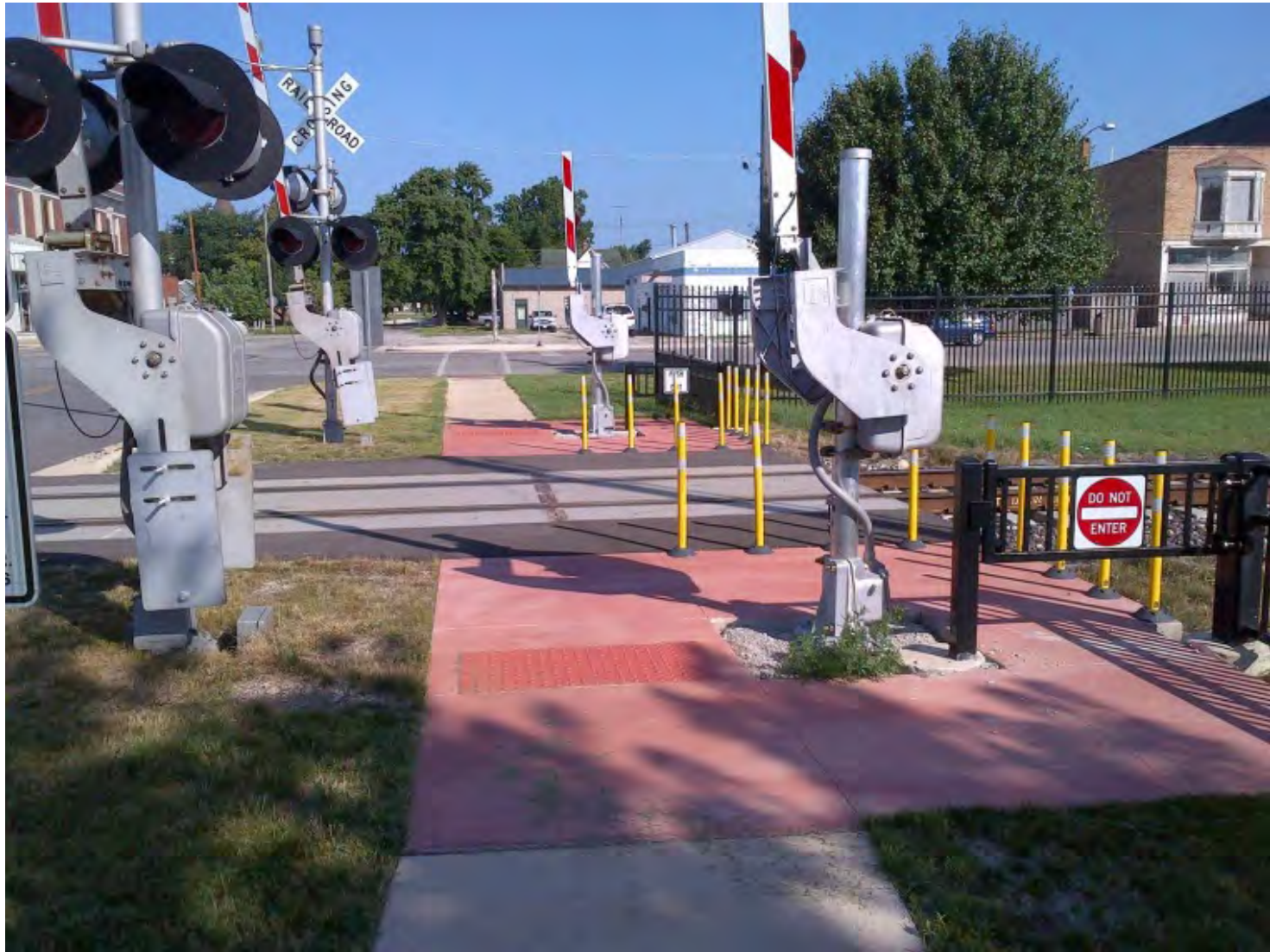
Typical pedestrian rail crossing installation
