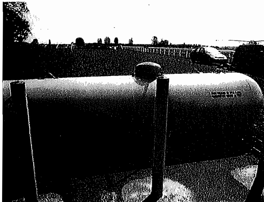
A 2000-gallon-water-capacity stationary ASME container is prohibited on the roof of a building.
