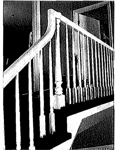
Transition from handrail to guard
