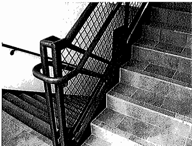
Interior exit stairway
