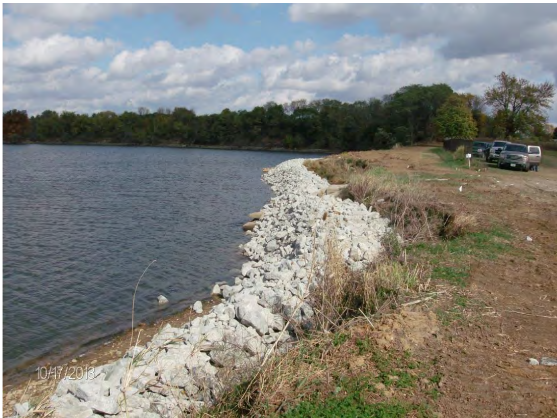
Shoreline protection near the Comlara Park Swimming Area
