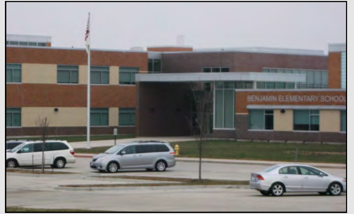
Benjamin Elementary School Grades K-5; 2013-14 enrollment: 590 McLean County Unit 5 School District
