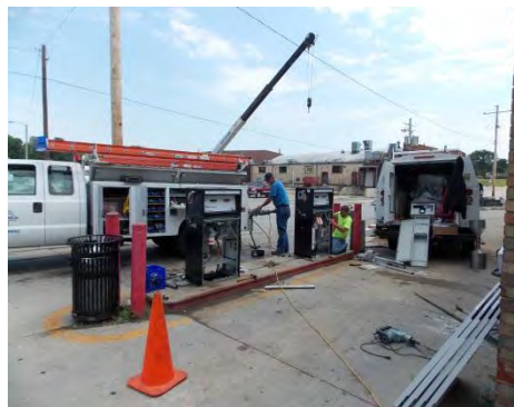
Old Fuel Pumps Removal
