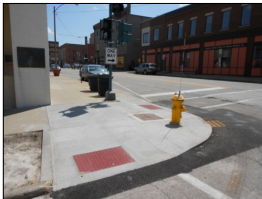
Figure 6: Example of Completed Inlet Repair Work
