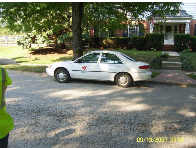
Kenyon Ct Before CRF Treatment in 2007
