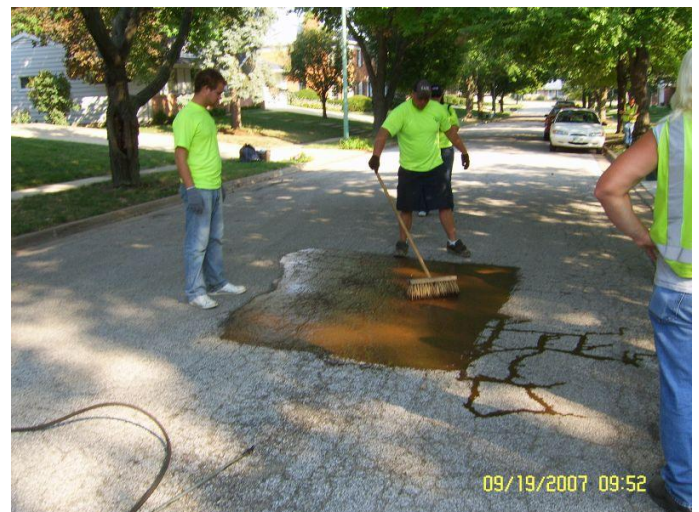
CRF Applied By Hand Applicator Then Broom Finish
