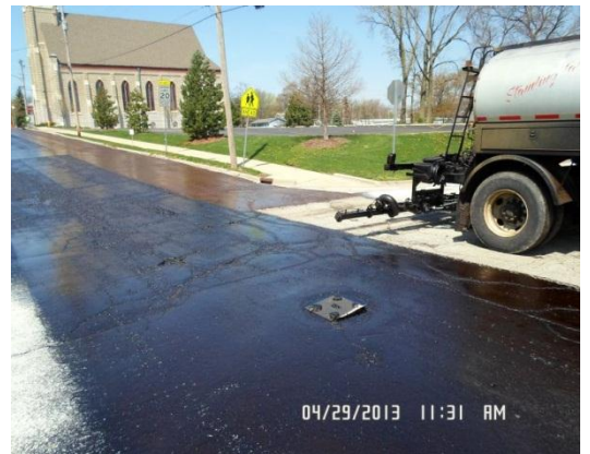
CRF Applied to North Side of Jackson Street
