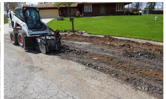
Street Division grinding crew milling asphalt on Heather Hill Road
