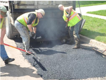
Street Crew putting hot asphalt down on Kenneth Drive
