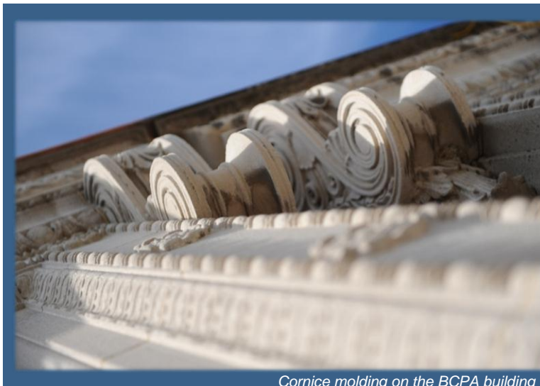
Cornice molding on the BCPA building
