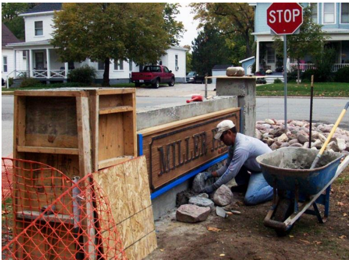
New sign installation at Miller Park
