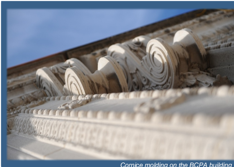
Cornice molding on the BCPA building
