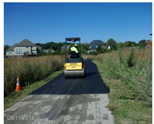
Asphalt replacement for portions of Constitution Trail
