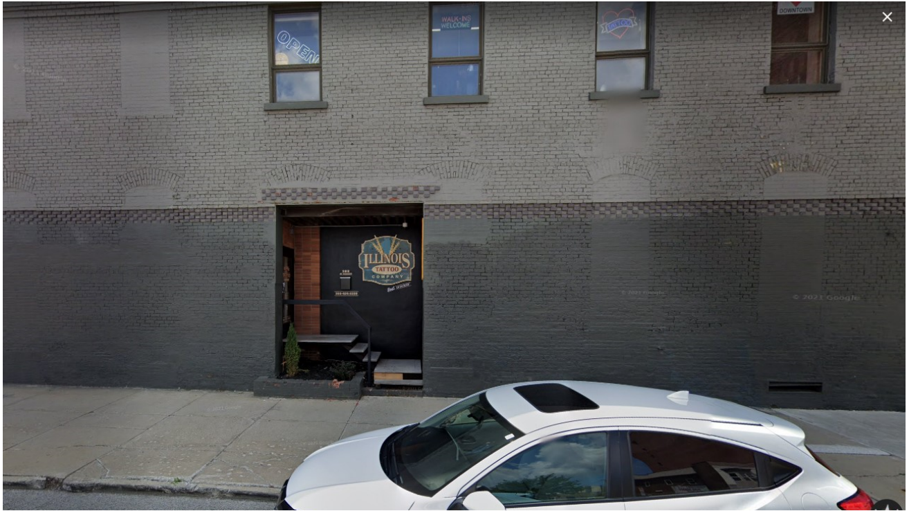
Attachment 3- Ground-Level View of 102 W Market Street
