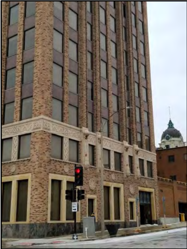
Figure 9 North elevation of the State Farm building.
