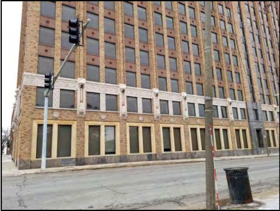
Figure 5 South portion of east elevation.
