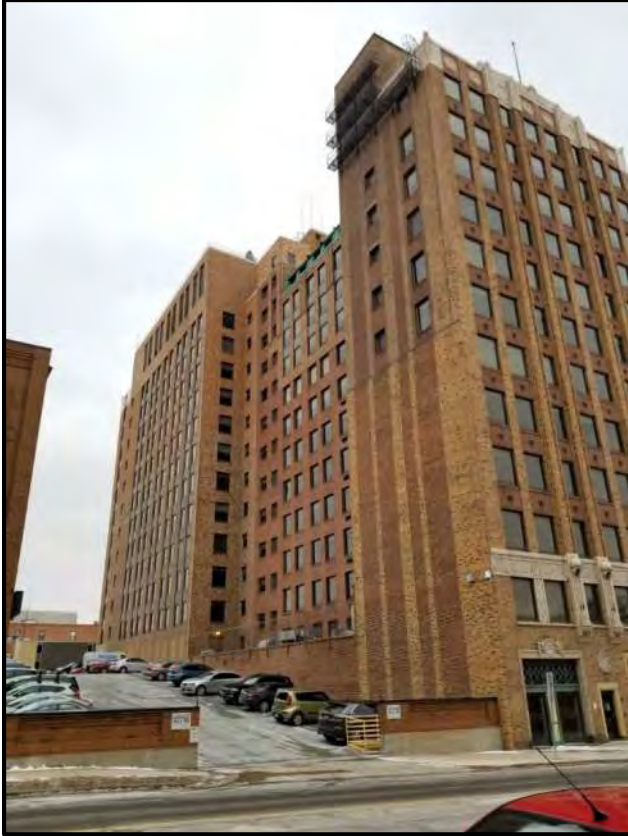
Figure 4 West Elevation of the State Farm building.
