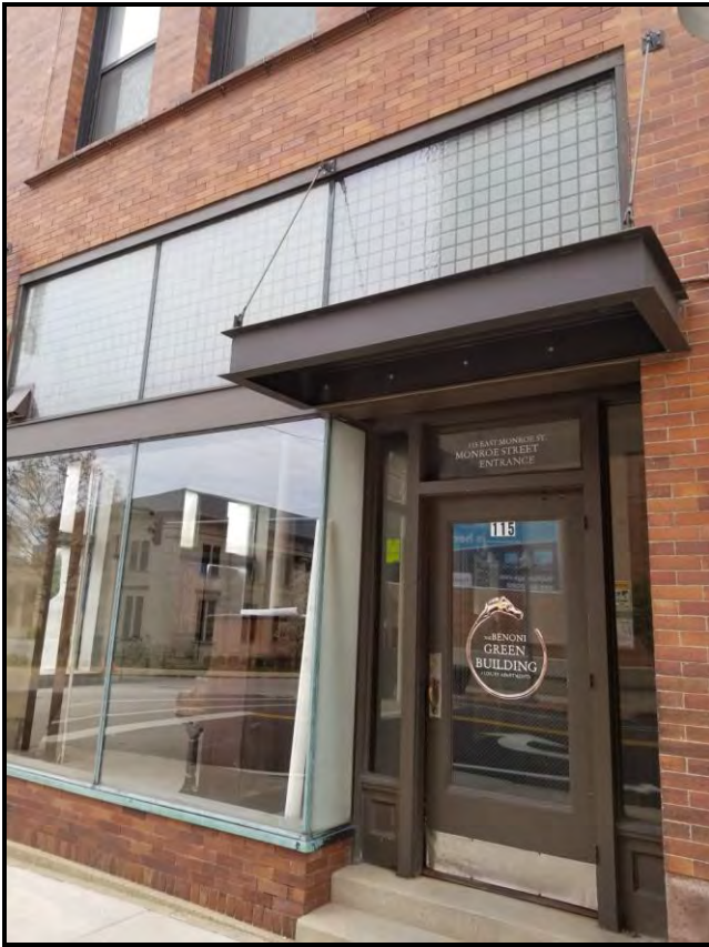
Figure 4 Front entrance on north elevation facing E. Monroe Street.
