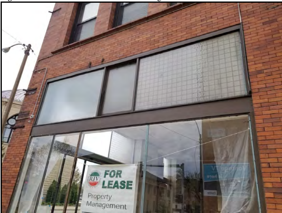
Figure 5 Transom windows on north elevation of 115 E. Monroe St.
