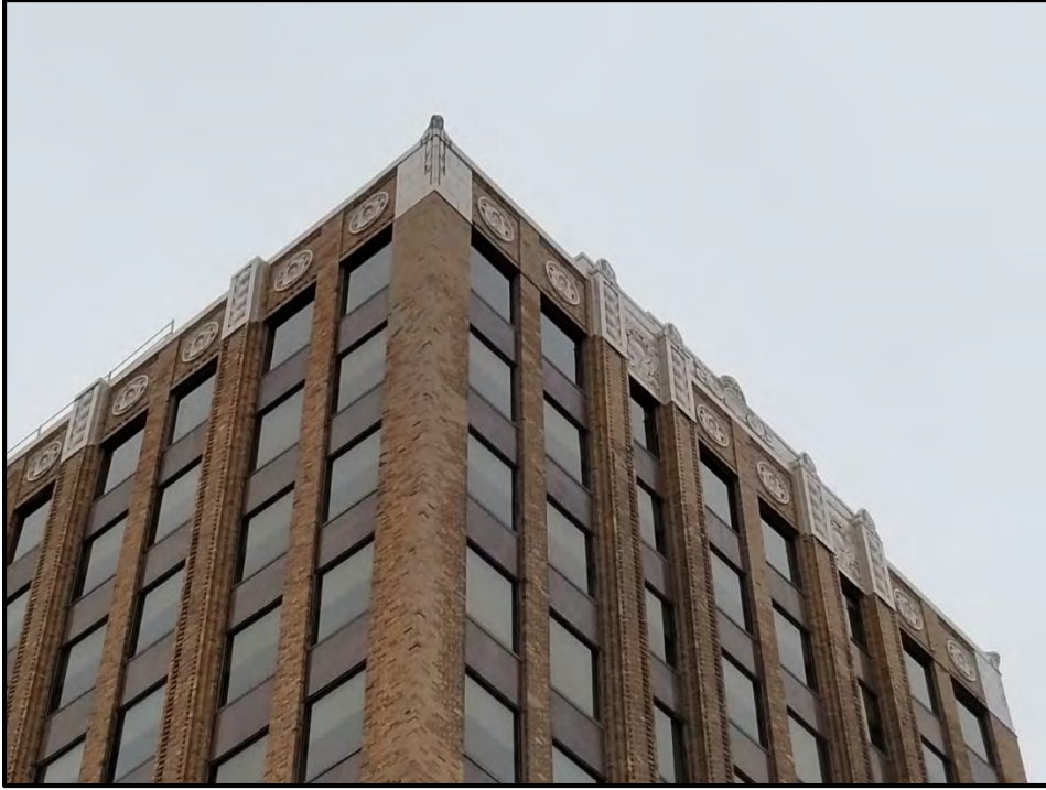
Figure 8 Northeast corner of the building showing the detailed cornice.
