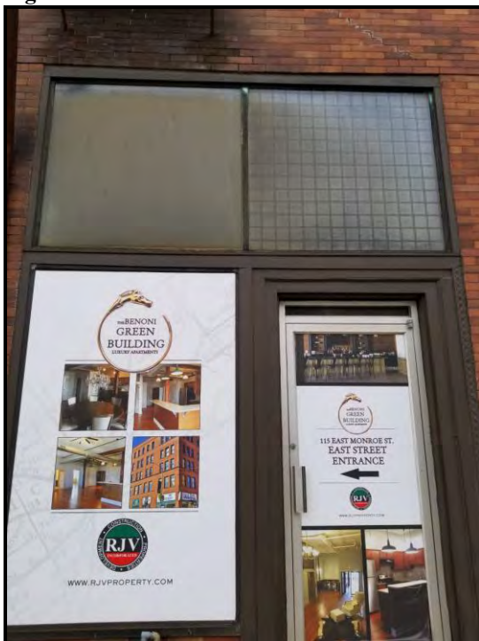
Figure 9 Door and transom windows on east elevation.
