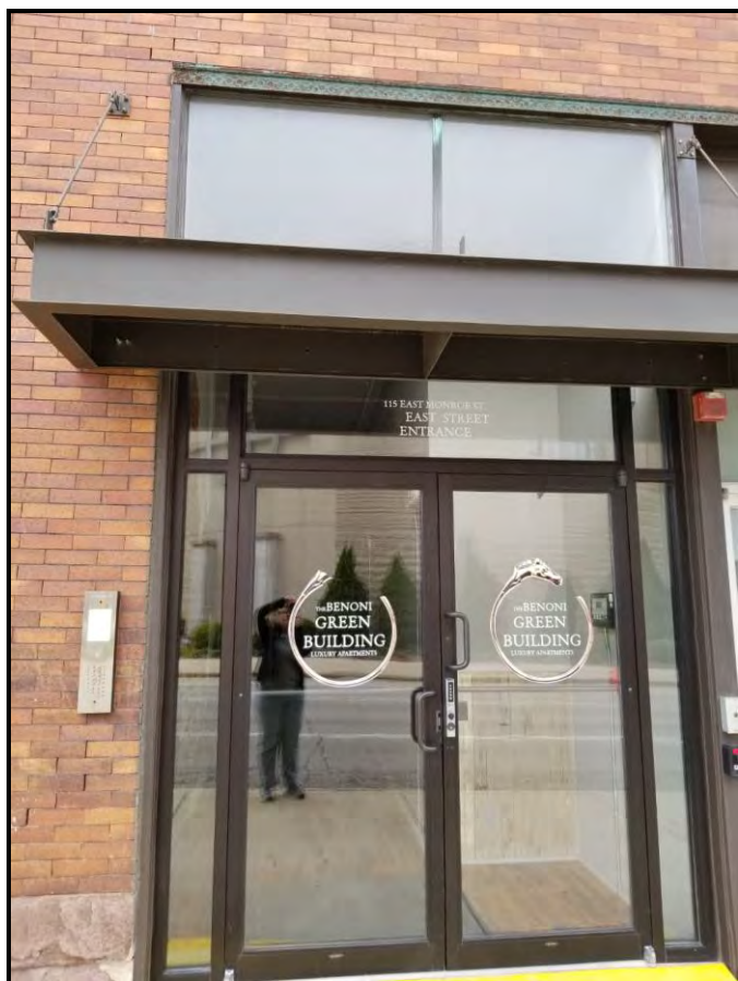
Figure 10 Entrance and transom windows on east elevation.
