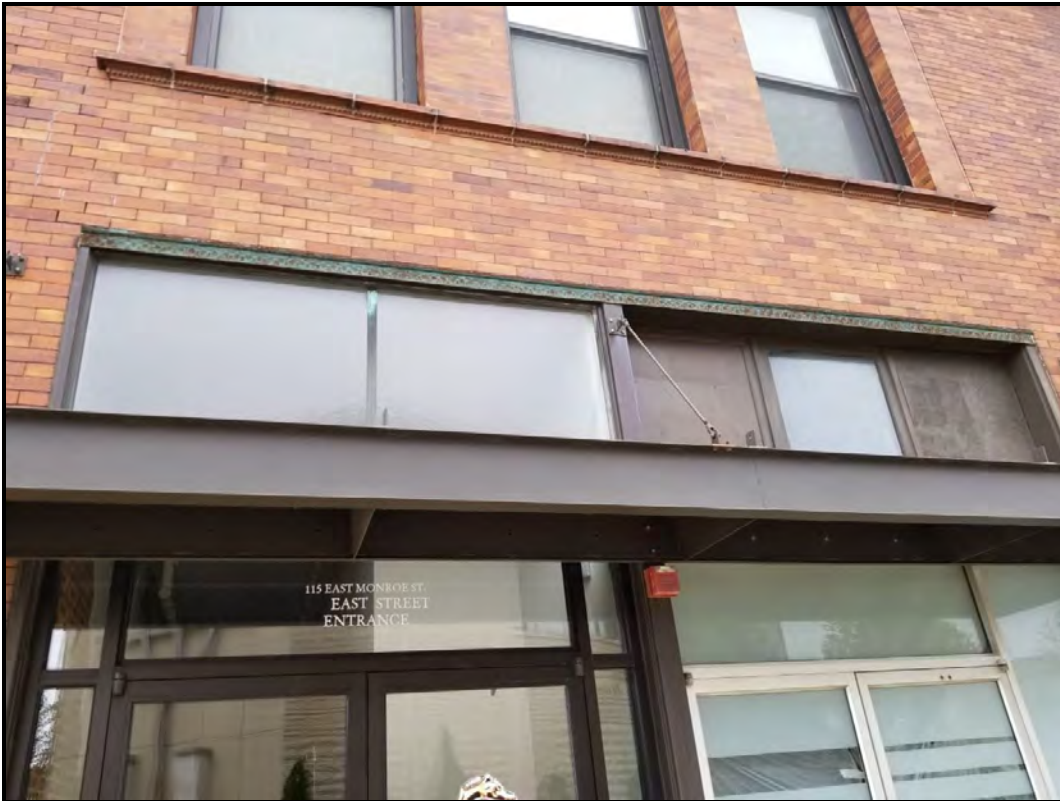
Figure 12 Transom windows above doors on the east elevation.
