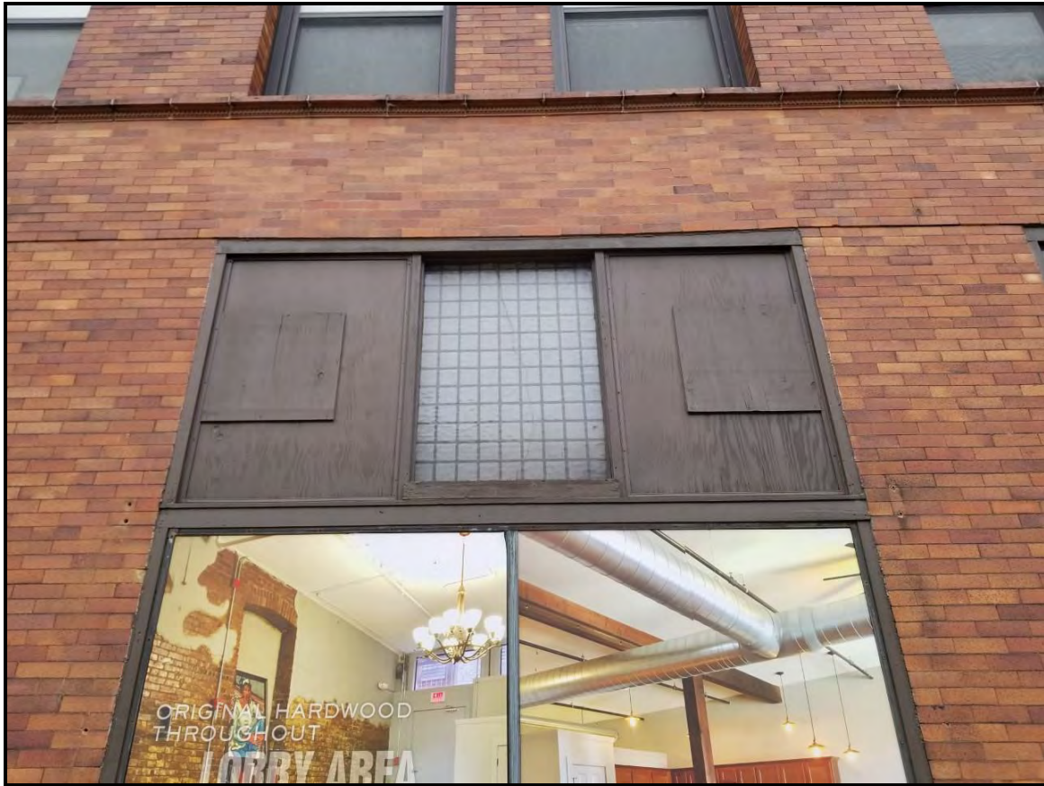
Figure 8 Transom windows on east elevation.
