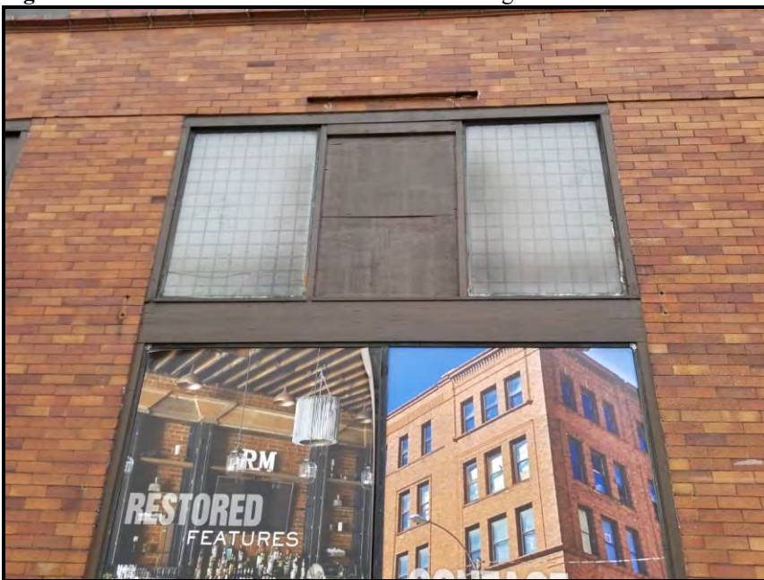
Figure 7 Transom windows on east elevation.
