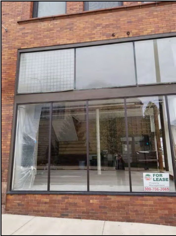
Figure 6 First floor windows on east elevation facing N. East Street.
