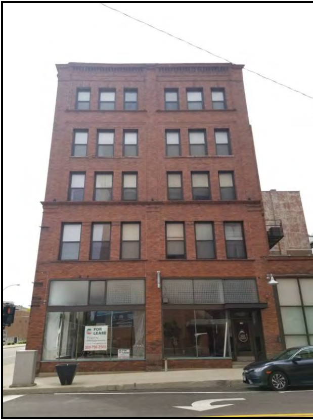
Figure 2 North elevation of 115 E. Monroe Street.
