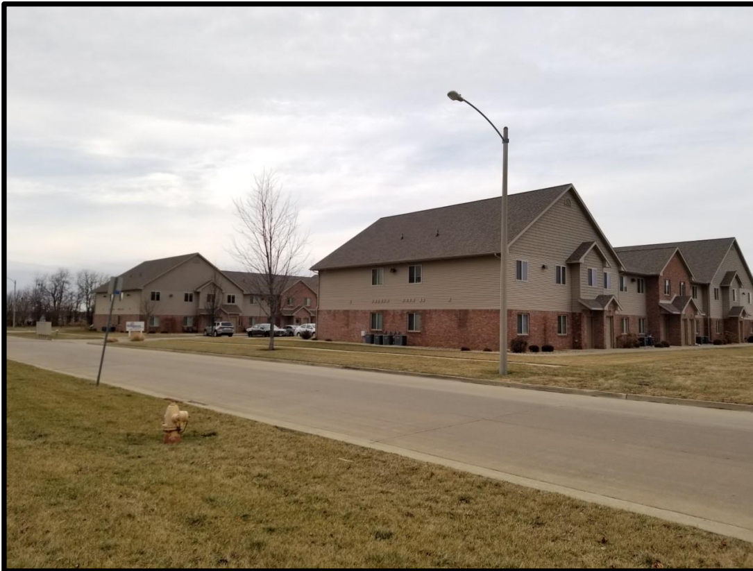
Figure 4 Multiple family residences on 3204-3212 Gerig Drive.
