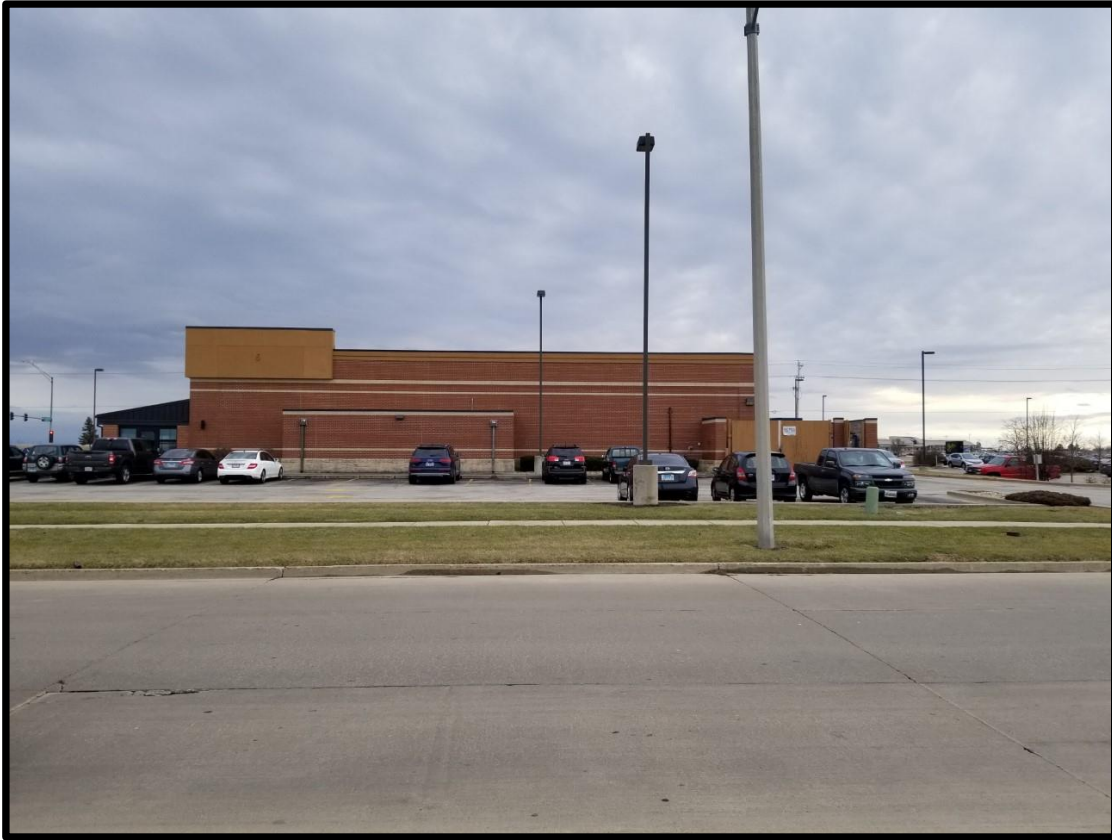
Figure 11 Rear elevation of Buffalo Wild Wings from Gerig Drive.
