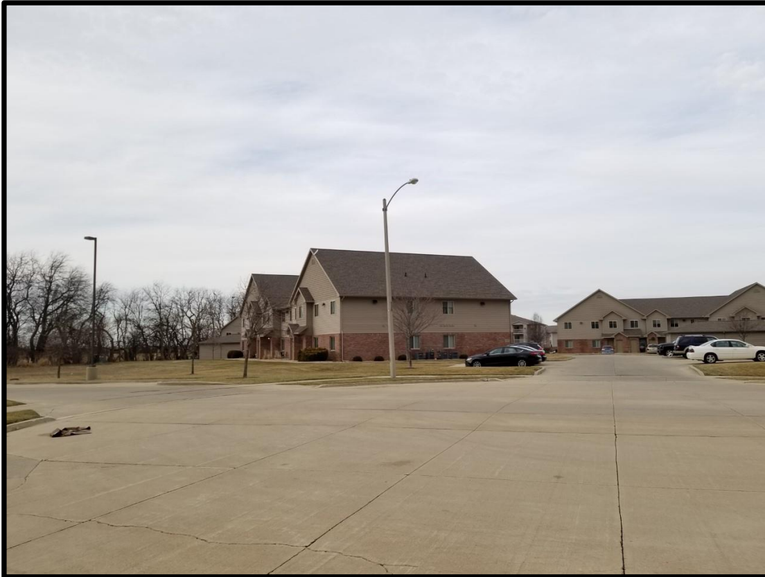
Figure 7 Multi-family residences at 2304 Gerig Drive.
