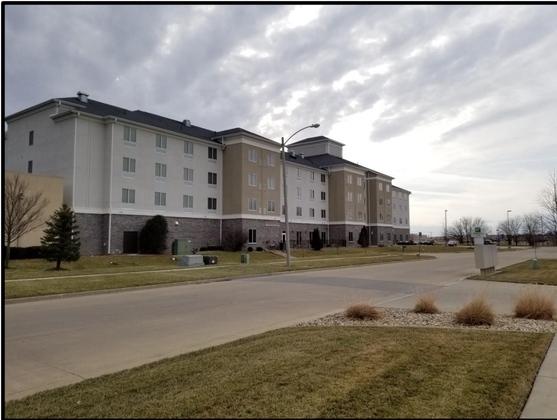
Figure 6 The rear elevation of Holiday Inn from Gerig Drive facing E. Empire Street.
