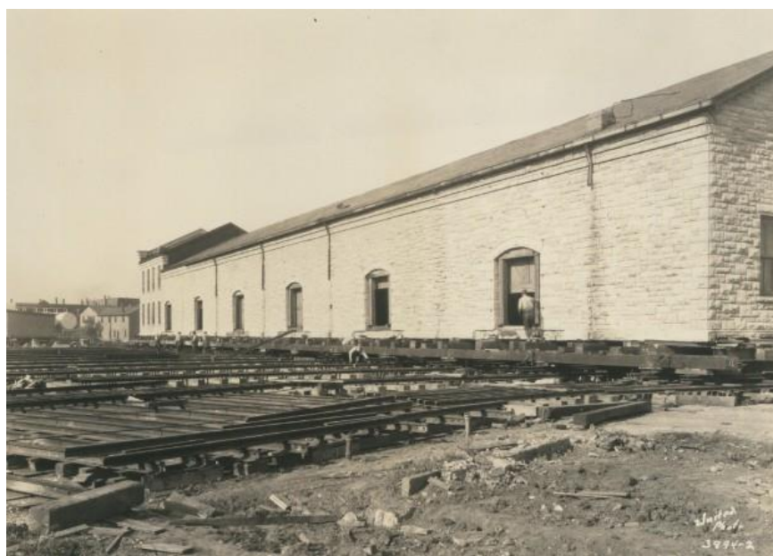
Visible in this photograph is the intricate system of rollers and rails needed to move the massive Chicago & Alton Railroad freight house to its new location in the summer of 1926. (Photo courtesy McLean County Museum of History).
