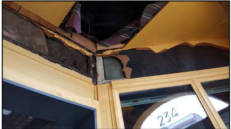
Inside the vestibule showing covered windows and glass
