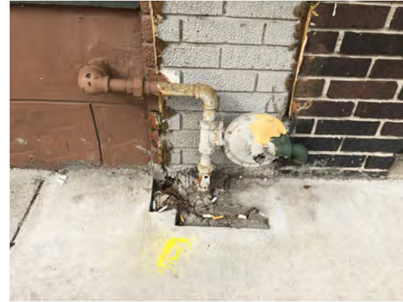
EXISTING GAS REGULATOR EXPOSED DURING INVESTIGATIVE DEMOLITION. SIDEWALK TO BE REPLACED.
