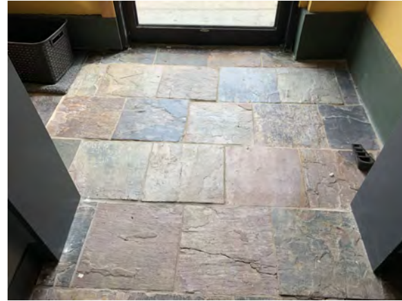
VIEW OF EXISTING VESTIBULE FLOORING AND WALLS TO BE REMOVED.
