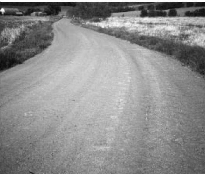
▲ New cold mix surface.
