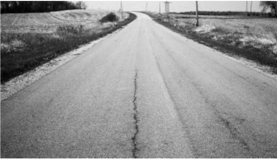
▼ Slight rutting; patch in good condition.
