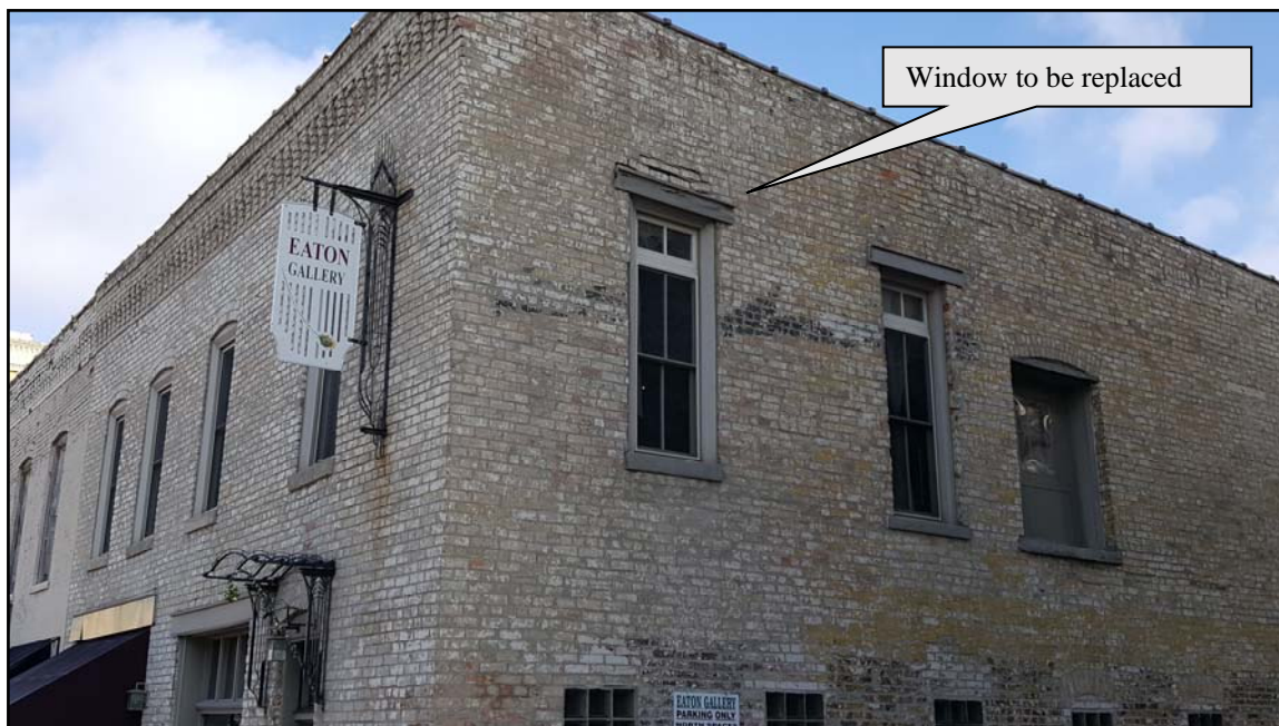
View from Center Street heading north toward the site
