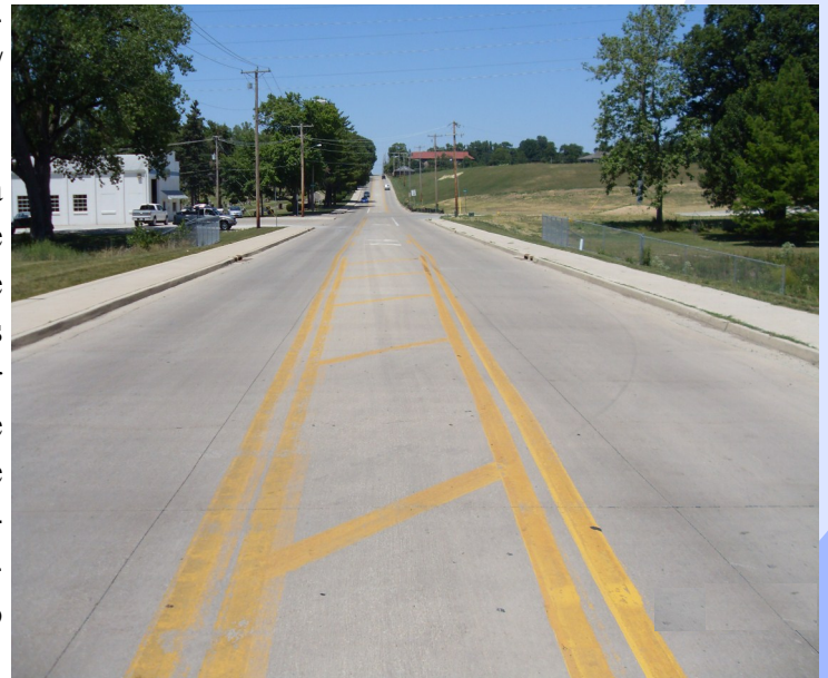
Previously completed section of Morris Avenue with wider lanes and bi-directional turn lane. This design will be extended to southern portions of Morris Ave.
