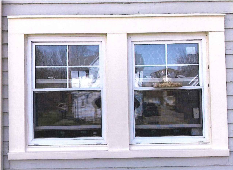
Detail of metal casing:
