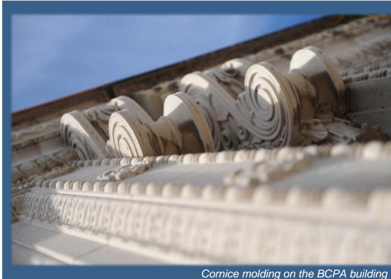
Cornice molding on the BCPA building
