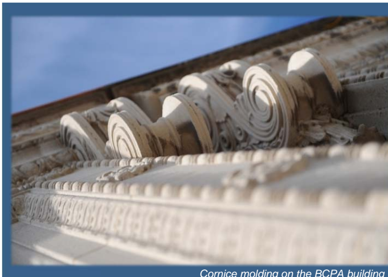
Cornice molding on the BCPA building
