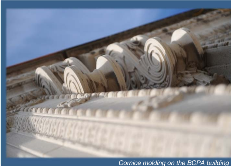
Cornice molding on the BCPA building
