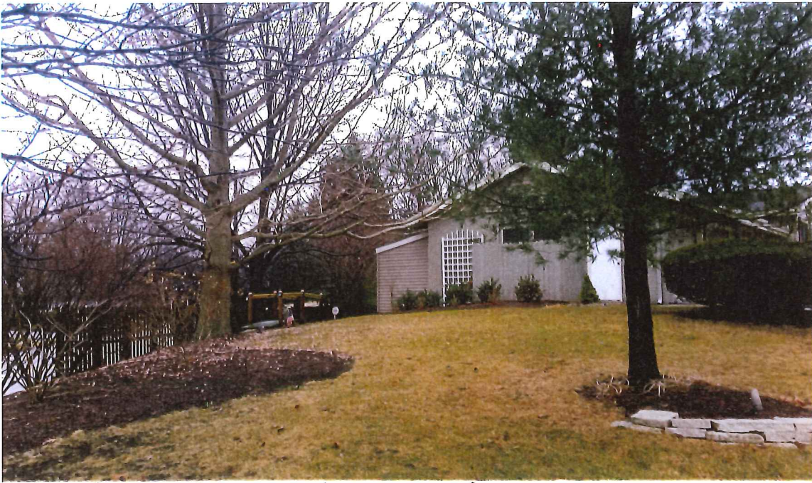
View from Cul de Sac toward existing GARAGE
