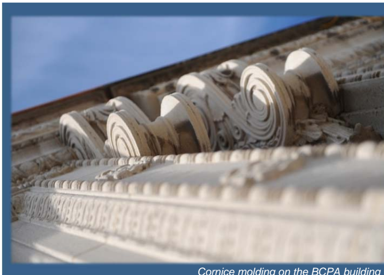
Cornice molding on the BCPA building
