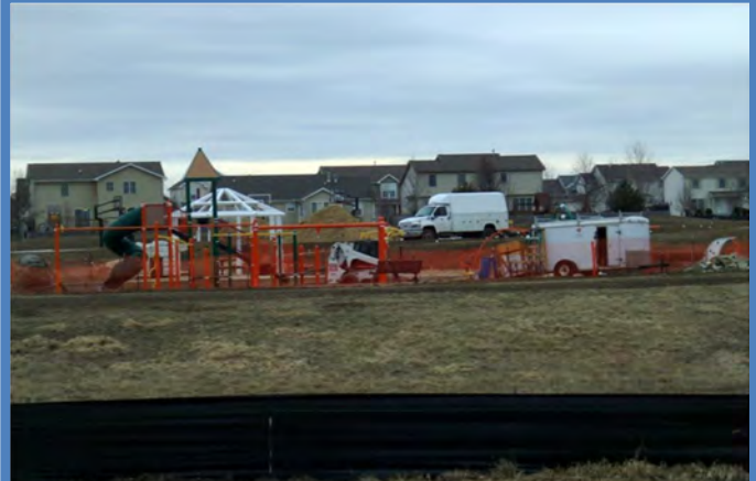
Playground installation at Gaelic Park
