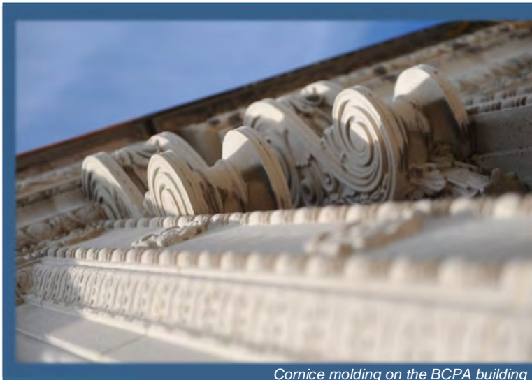
Cornice molding on the BCPA building
