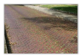
Figure 18: Effects of driving on vegetation between bricks
