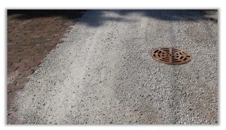
Figure 16: Temporary gravel patch
