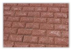
Figure 14: Brick-stamped concrete
