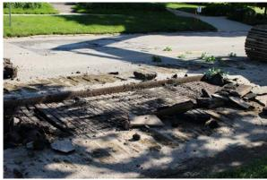
**3.** Clean residual asphalt from the bricks. Power washing is a common method.
