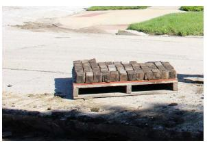
**6.** Carefully stack undamaged bricks on a pallet on location or at another location, depending on the method used. Count on having to discard 30 percent of the bricks because of various types of damage.
