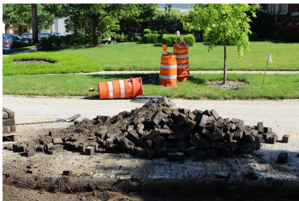
5. Once the bricks are removed, place them in a pile on the nearby road so that they can be palletized. Alternatively, haul them away to another location to be palletized later.
