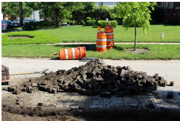
5. Once the bricks are removed, place them in a pile on the nearby road so that they can be palletized.
