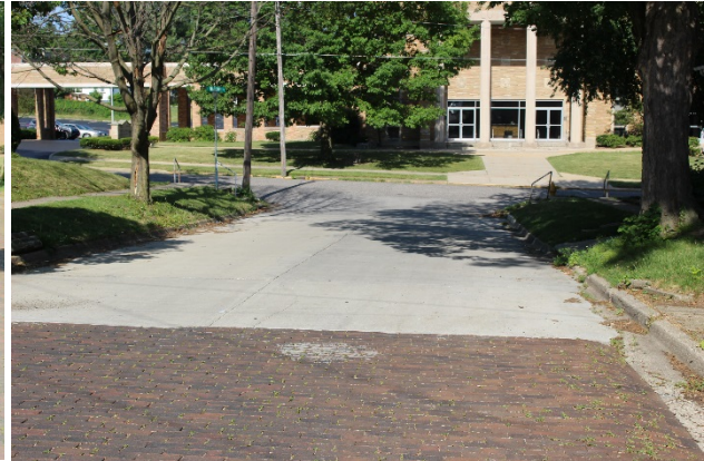
Figure 8: Concrete portion of Elm St., from Center St. to Madison St.
