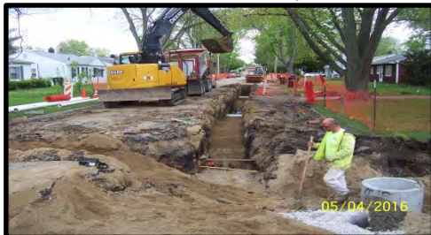
Start of Construction Ryan Drive.
