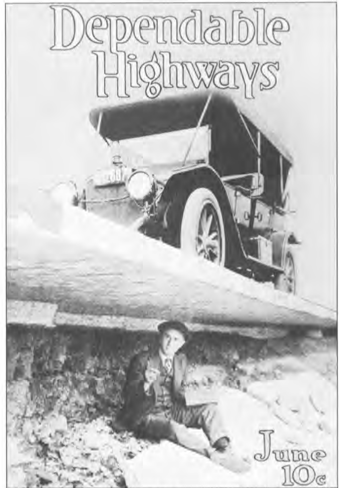
Above: Dependable Highways, the magazine of the National Paving Brick Manufacturers Association, heavily promoted brick paving from 1916 to the 1920s. This June 1916 cover photograph left no doubt about the strength of a monolithic brick paving system. Below left: This advertisement for the Danville Brick Company appeared in the April 1917 issue of Dependable Highways.
