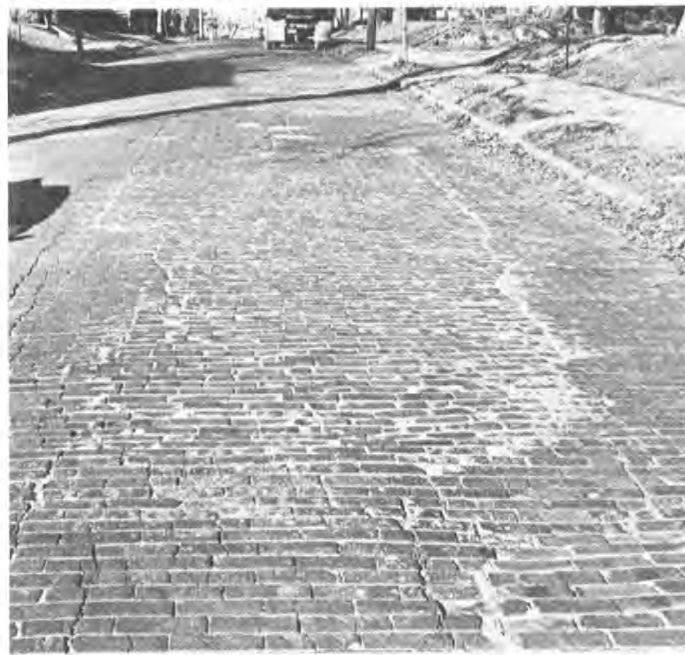
Above: This patch was pictured in a 1916 issue of Dependable Highways . The repair technique is virtually the same today. Below: This brick pavement in the Belleville Historic District was recently patched and sand filler installed.
