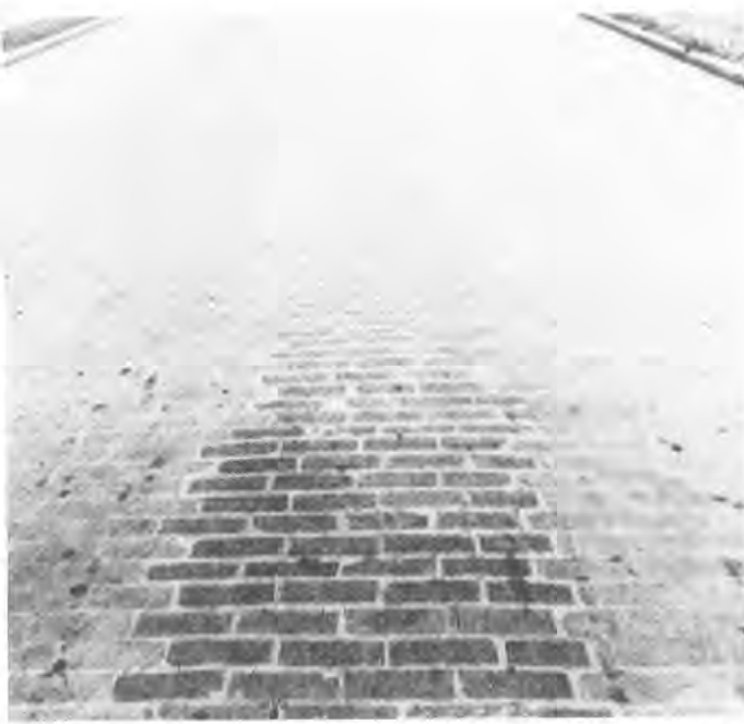
Above: This patch was pictured in a 1916 issue of Dependable Highways . The repair technique is virtually the same today. Below: This brick pavement in the Belleville Historic District was recently patched and sand filler installed.
