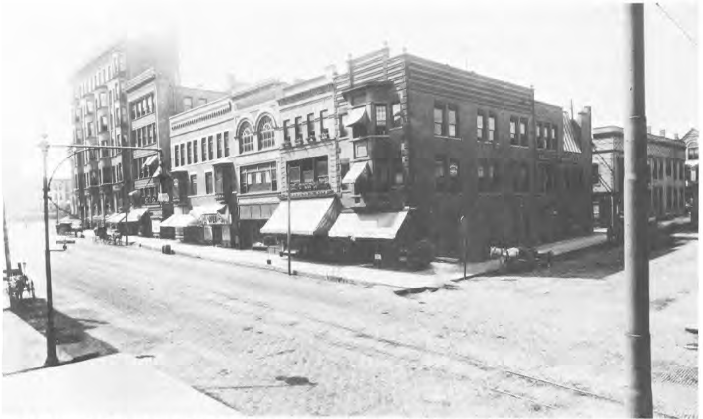
Note the herringbone pattern at the intersection and straight pattern for the block fronts on turn-of-the-century Main and Monroe streets in Bloomington. Photo: McLean County Historical Society
