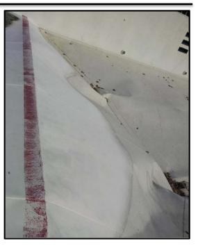
paint job is needed to preserve the pool. The bare aluminum walls will corrode if not painted. Multiple tears in Holiday's pool floors were discovered and the extent of repairs is unknown, a new pool liner may be required as part of the repairs.
