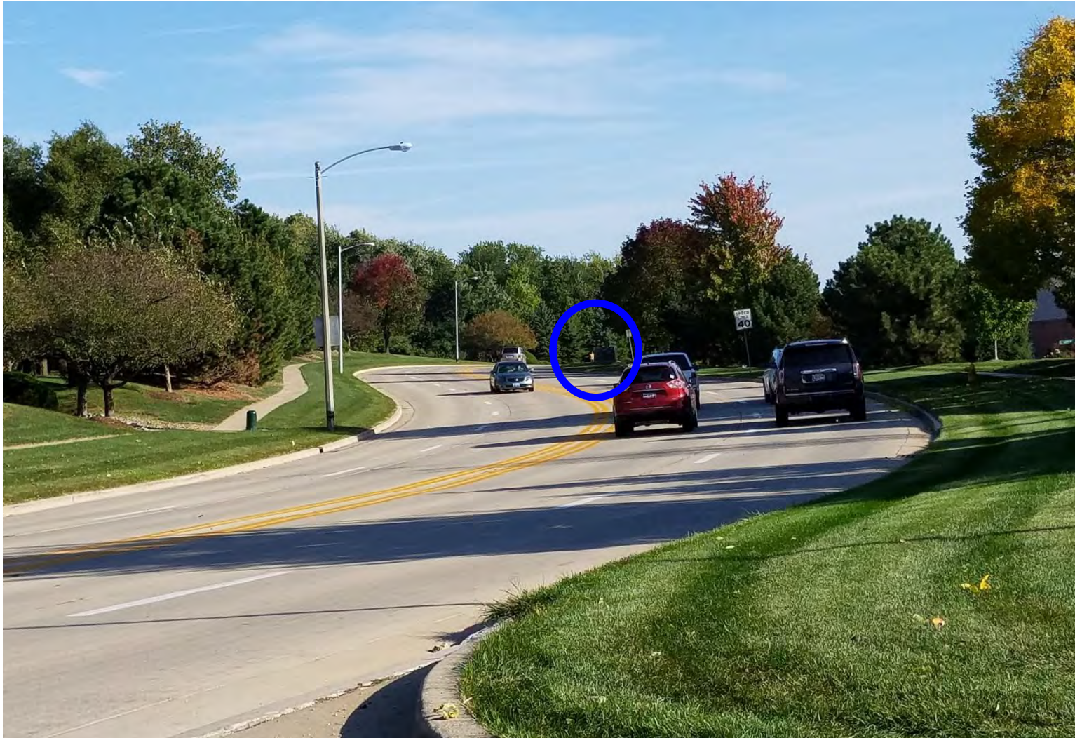
Photo 9: Looking Right to 870 feet (MAX distance of continuous sight = PC @ ~74 mph, MU @ ~48 mph)
