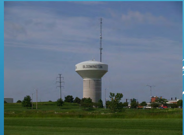
Hamilton Tank Valve Reconstruction
