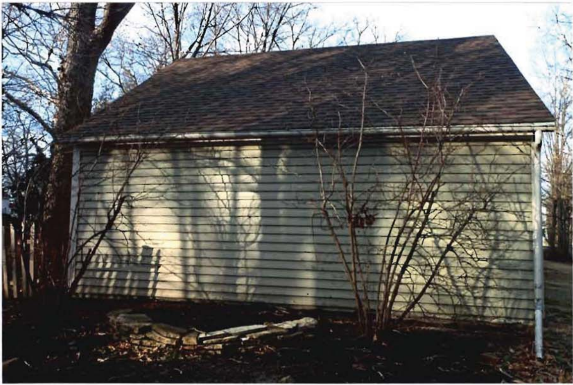
South Side of garage
