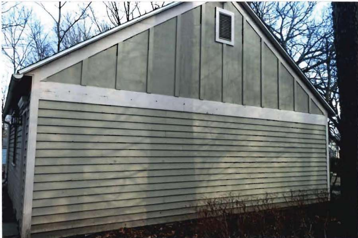
West side of garage
